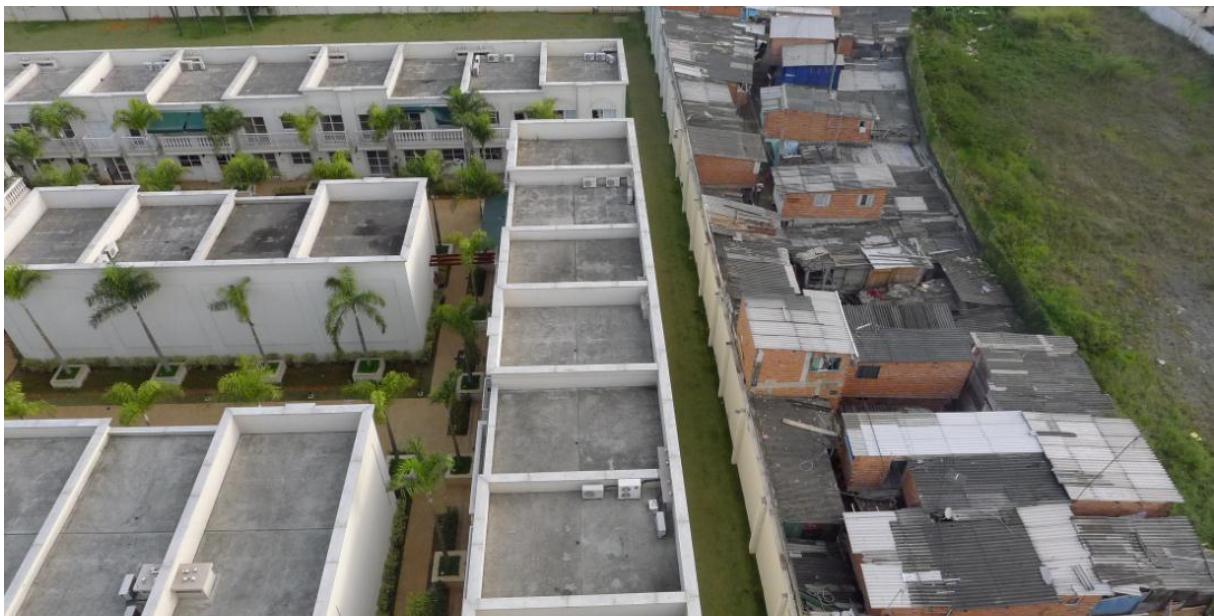
Picture 4: The wall separated the corporate offices to a favela , Vila Leopoldina
